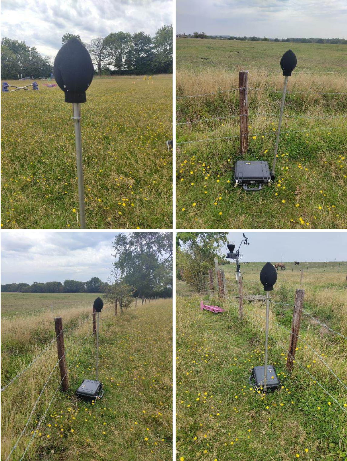
Figure 14.2-19: Photos of Equipment at NML09
